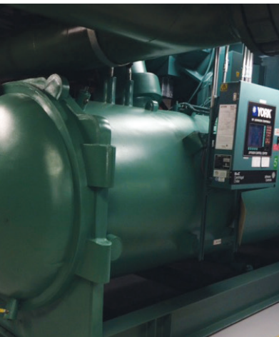
YORK® variable speed drive YK centrifugal chiller.
