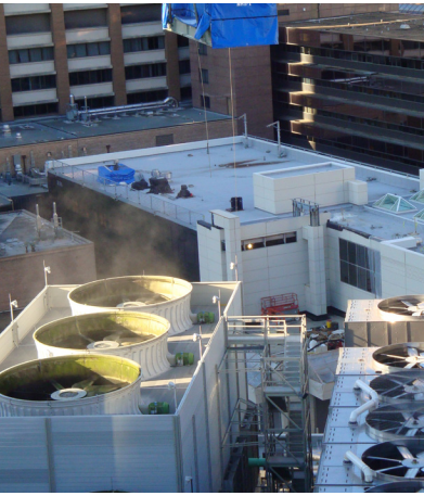
Bird's eye view of the central utility plant.
