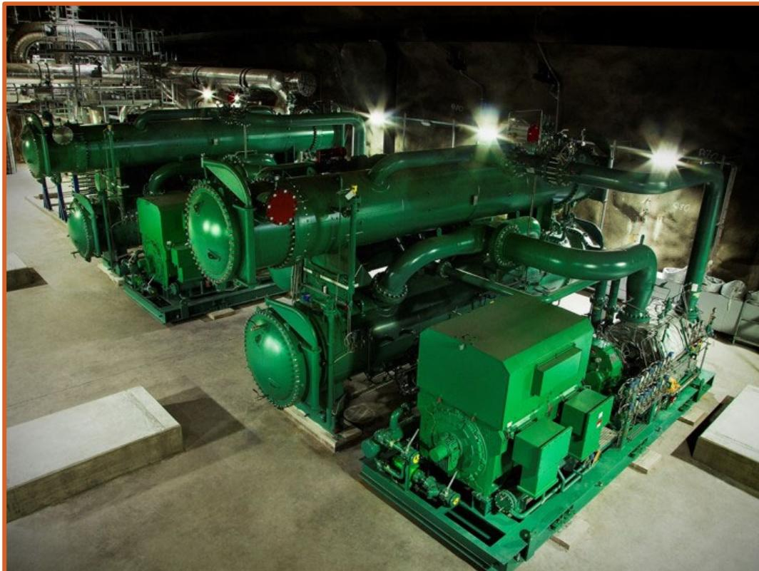
Helen's investment in two massive centrifugal heat pumps in 2018, resulting in less usage of fossil fuel (coal) and cutting CO<sub>2</sub> emissions by 20,000 tons per year
