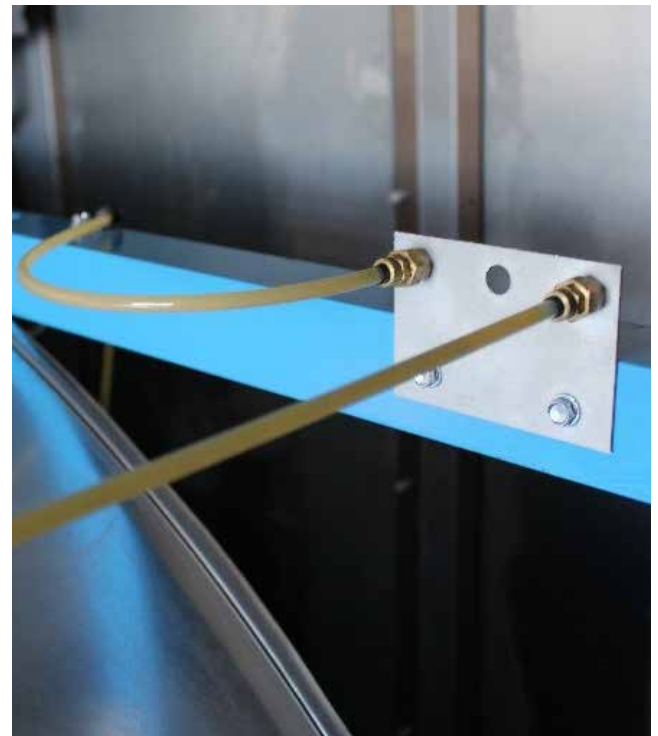
Figure 53: Grease Line Connection Mounted on Fan Frame
